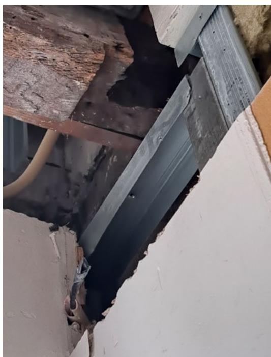
31. Adjustment of wooden construction due to subsidence (Photo: Vera Kuijpers)
