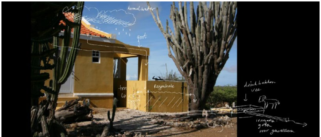
10. The principle of rainwater collection and distribution system of the Bonairean Landhuis Rooi (Photo: Jet Bakels. Edited by LILA Living Landscapes)
