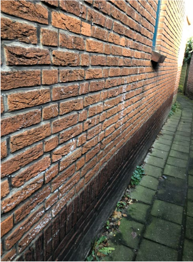
32 Frost damage to bricks due to rising damp
