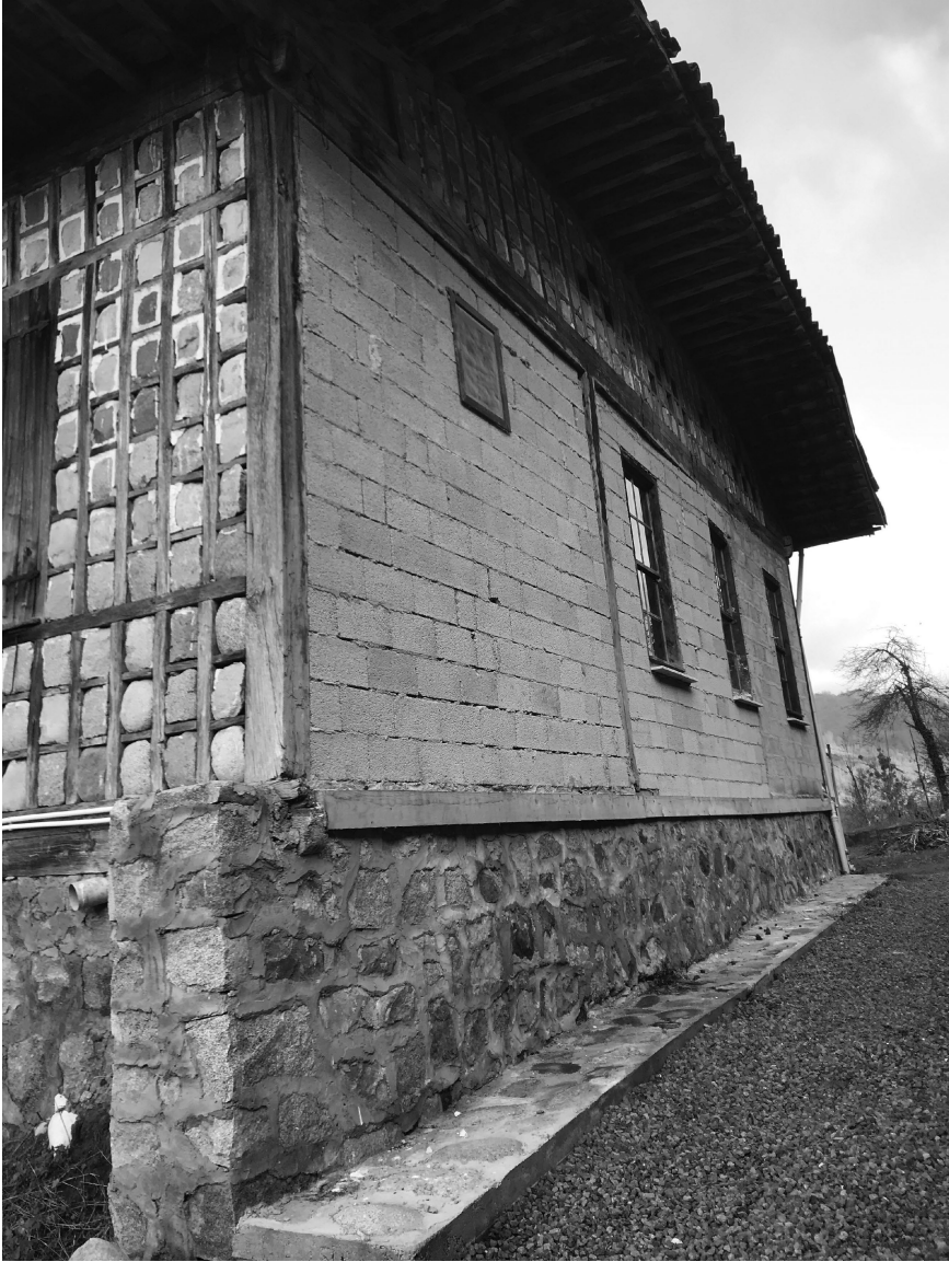
Figure 5.8 The degradation of the rear façade of the Ş.A. House due to landslides in Çağlayan Village in Fındıklı of Rize.
