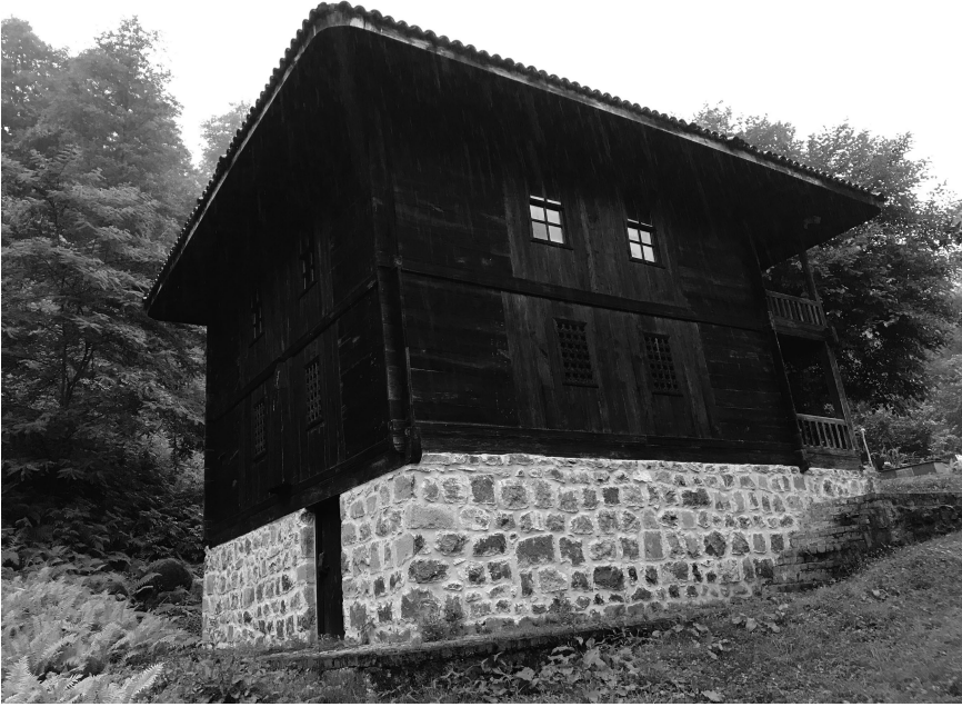
Figure 3.2 Wooden masonry (yontma yığma) construction system used in Meyvalı mosque in Findıklı. Photograph by the author.
