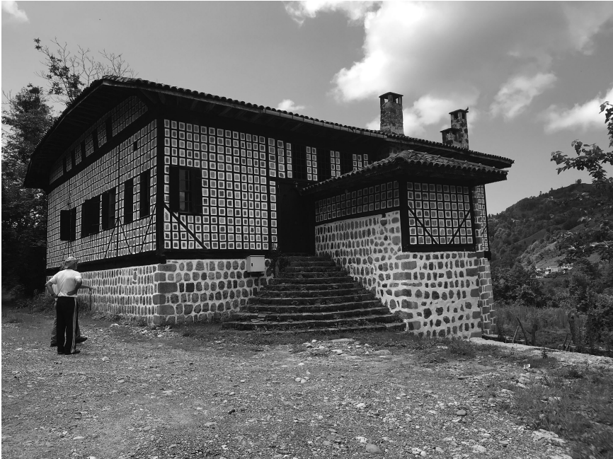
Figure 3.4 Cell-infilling is quite common in Fındıklı. Photograph by the author.
