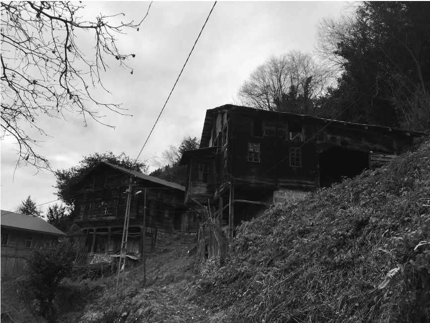
Figure 3.3 Wooden infilling construction system used in the vernacular houses in Çamlıhemşin. Photograph by the author.
