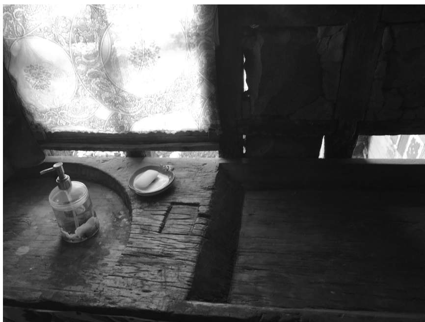
Figure 4.3 A wooden kitchen countertop for washing dishes and clothes in a vernacular house in Hara Village taken back to the 1830s. Water is carried to the washing area by wooden channels. Photograph by the author taken on July 3, 2019.
