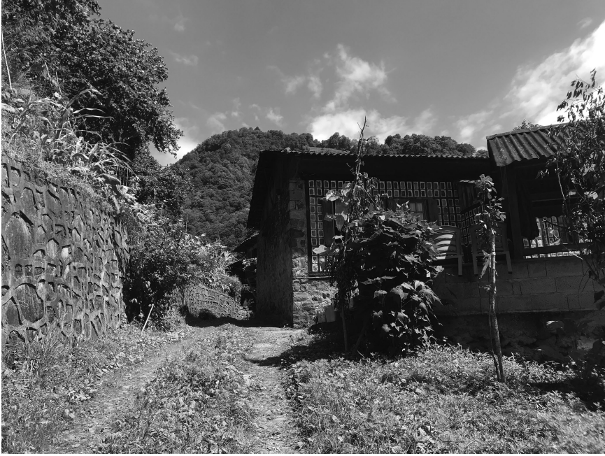
Figure 7.2 T.H. house is vulnerable to rock falls, which is why the rear façade was built with stone with no opening. Photograph by the author on January 11, 2019.
