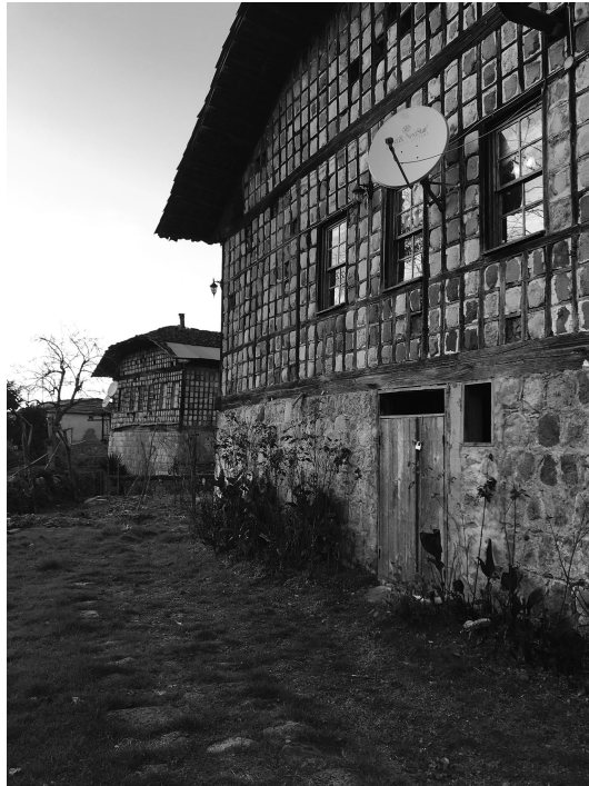
Figure 4.2 The low-pitched roof structure with extended roof overhangs is quite common in Çağlayan Village. Photograph by the author on January 12, 2019.
