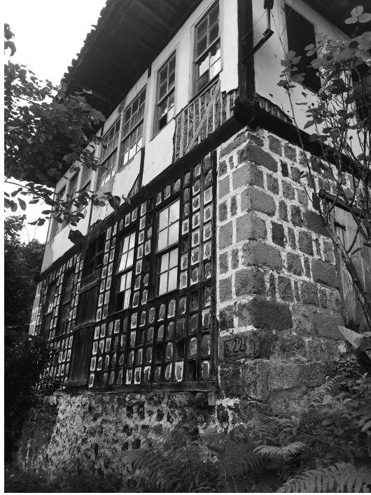
Figure 3.5 Combined construction system, including stone, stone-infilled timber, and çakatura on the top floor. Photograph by the author.
